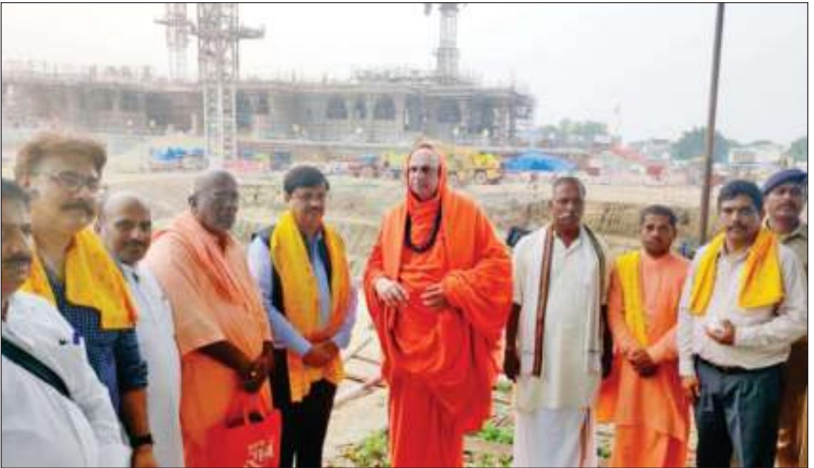
HH Jagadguruji after the darshan of Ramlalla at Ayodhya viewed the construction of Ram Temple there. Industrialist Sri Saurav Sharma, Sri S.P. Manjunath, Associate Secretary of VHP's Central Committee Sri Gopalji, Swamijis, officers and officials of JSS Mahavidyapeetha were present (July 12, 2023)
